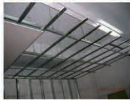
Furring C-Channel Ceiling System
