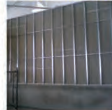
Board joints are staggered
